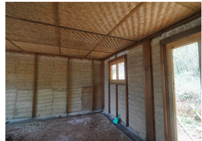
Prototype house construction at Kalapang, Mongar
