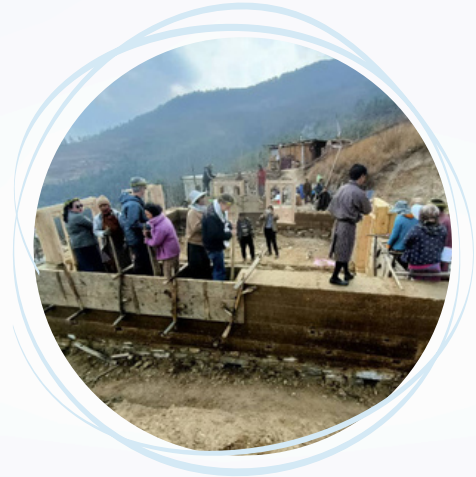
Prototype House Construction at Gomche, Paro
