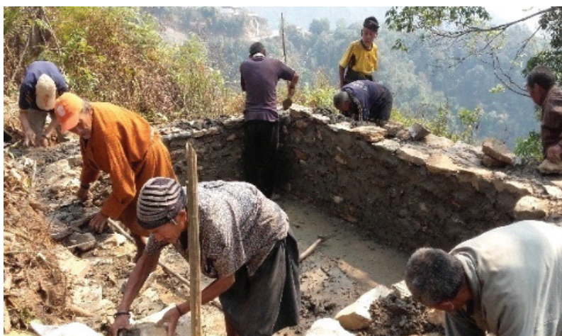
Water tank construction at Migkuri village, Pema Gatshel
