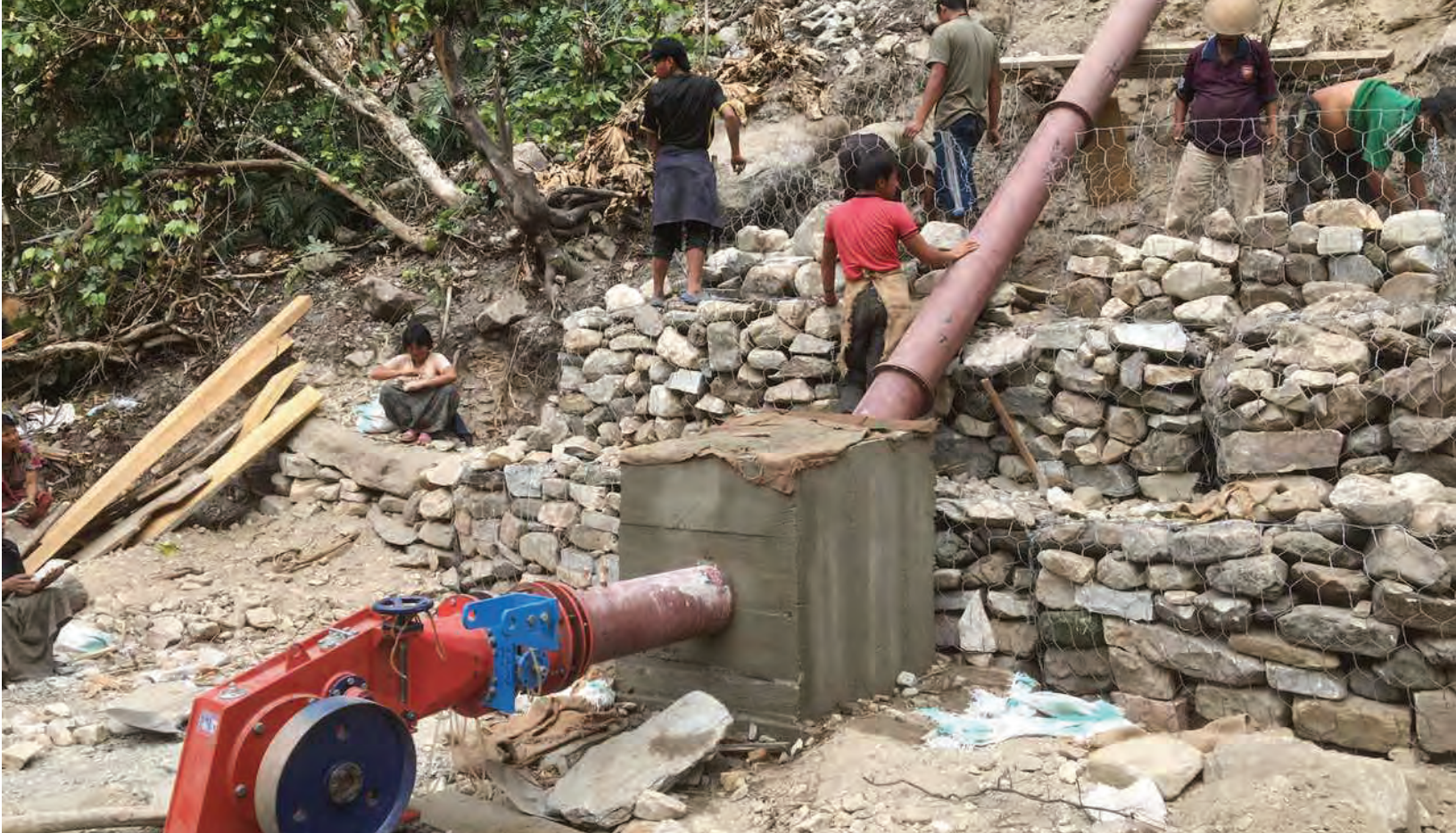
Micro Hydro project site in Dali, Zhemgang
