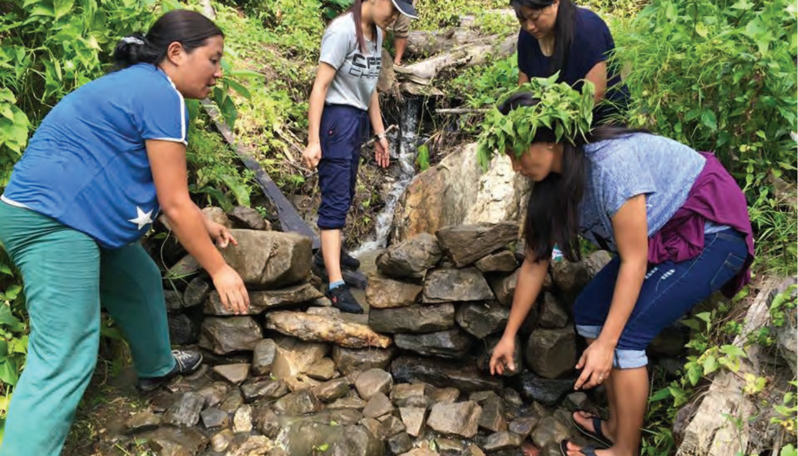
Communities learning construction of check dams using stones at Tsirangtoe, Tsirang
